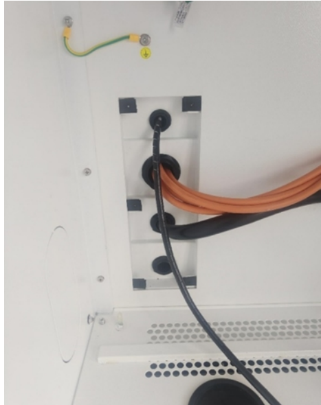
Figure 7-39 Panel ground cable installation
